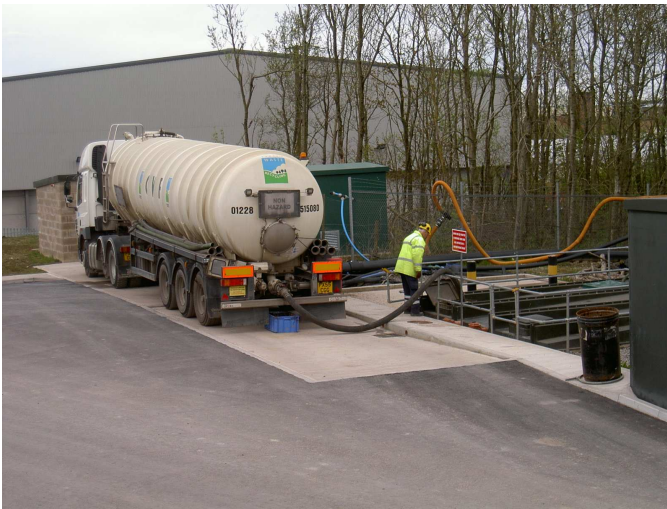
Core sampling of tanker for laboratory acceptance testing prior to treatment. Tanker discharging to LWTF reception tanks following satisfactory laboratory acceptance testing.
